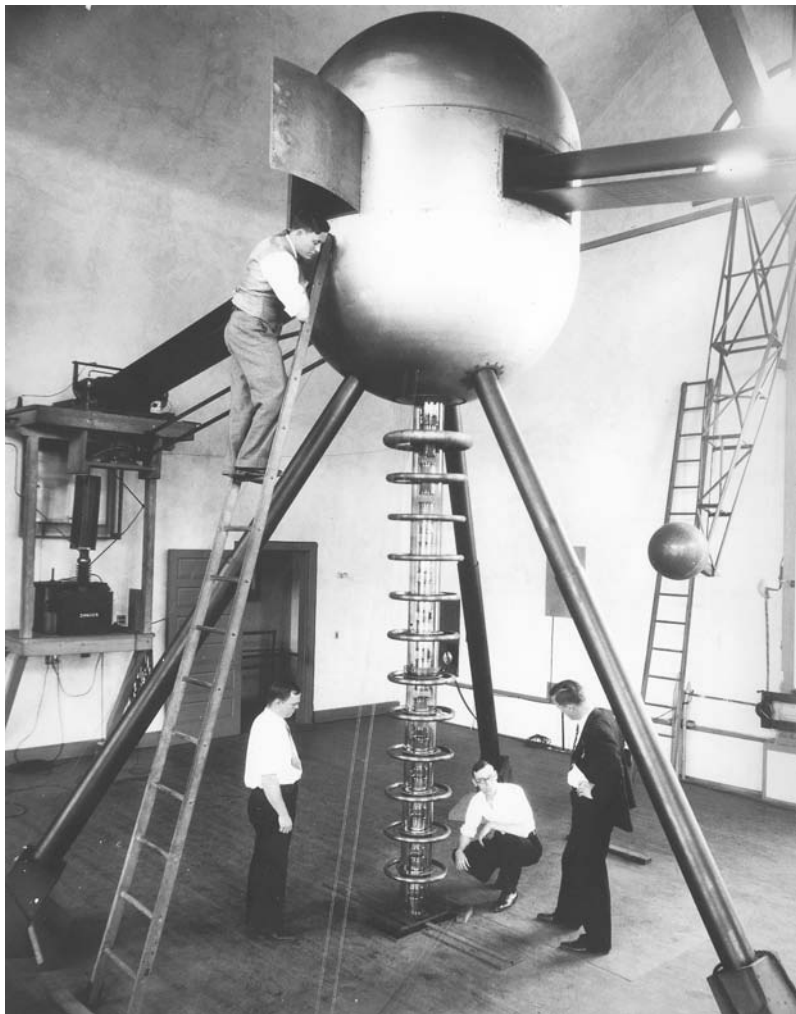
Figure 10.7. The completed two-meter generator, 18 May 1935. Dahl is on the ladder; on the floor (left to right), Meyer, Hafstad, and Tuve. DTM Archives 3662; Tuve, Hafstad, and Dahl, PR, 48 (1935), pp. 315–337, on p. 322.
